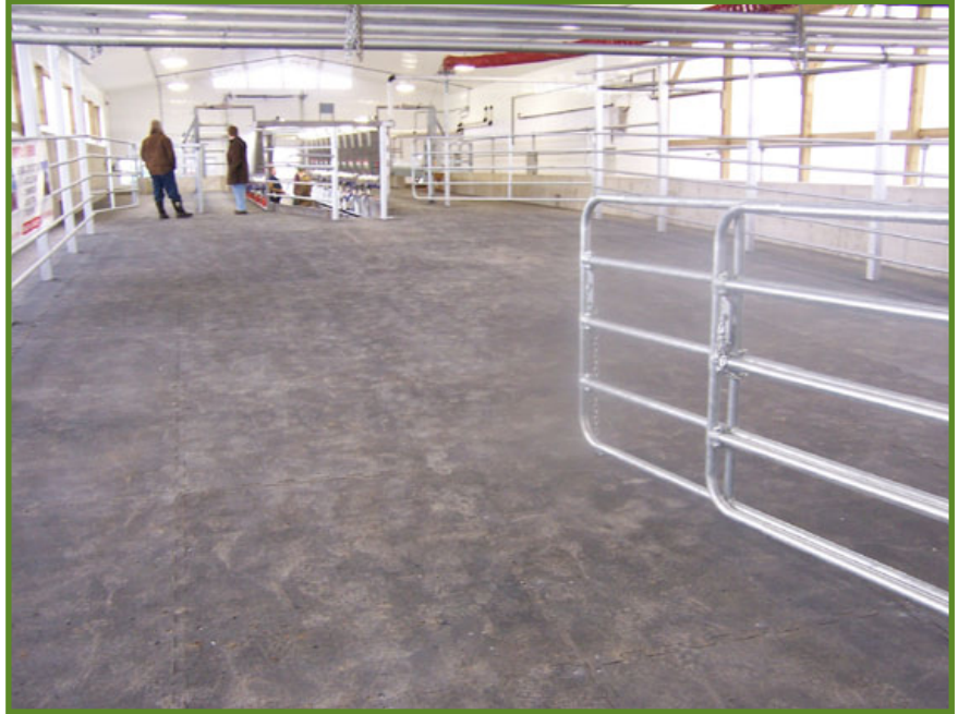
Solid coverage in a non-sand flush barn.
