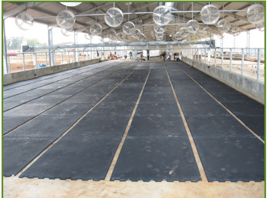
Mat strips in a sand-flush barn.
